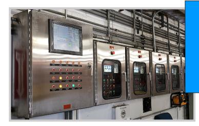
MurCal's municipal designs include a CENTRAL CONTROLLER which reads overall station sensors like wet level, system pressure and flow. The central controller COMMUNICATES with individual engine controllers using high speed CAN communications for reliable and timely control. It determines the least expensive operating mode by deciding which engine to start or by implementing a peak shaving strategy.
